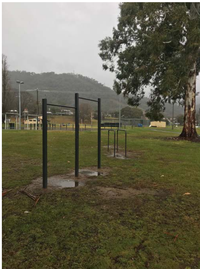
Figure 11: Mount Beauty- Existing equipment includes two static pieces. Lacking under-surfacing, with water accumulation after rain.
